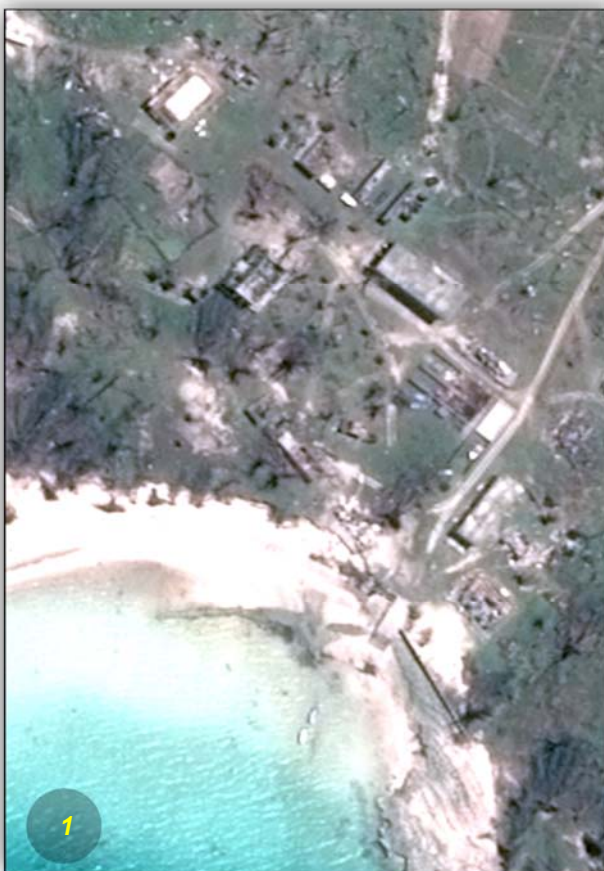
Post-Event-Image – Damaged Structures Pleiades - 22 April 2016 © (CNES 2016) - Distribution Airbus Defence and Space
