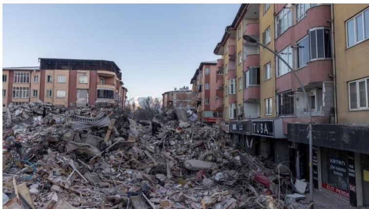
Figure 33. Collapsed structures in Elbistan, Türkiye.
